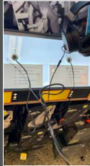
Messy wires and cables
